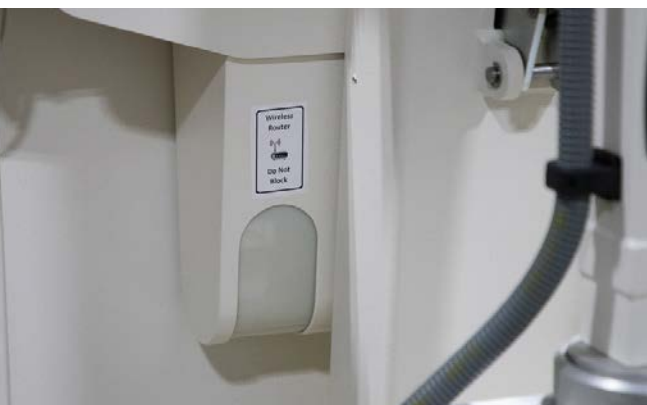
Water Tight Housing for Wireless Router
